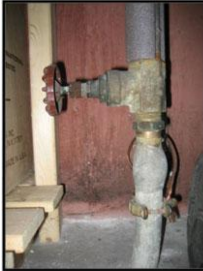
Lead service lines often have a "bulb" shaped connection. (3)
